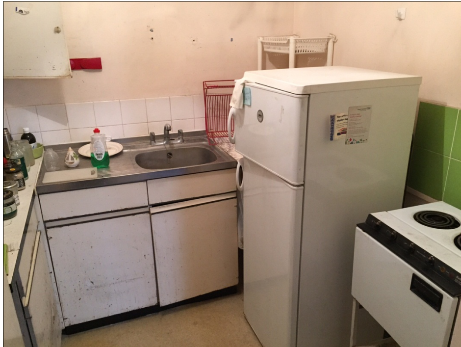
Photograph of Existing Housing (Kitchen):
